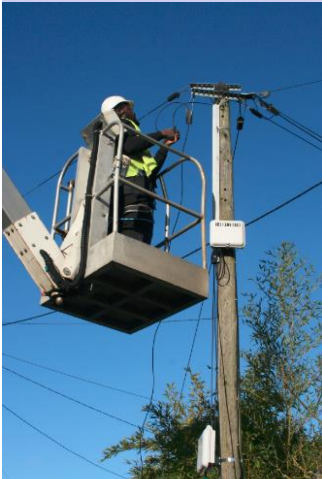
Appui FT en bois – PBO 3M
